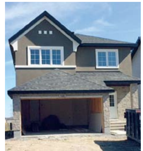
Sept 19: Stucco and stone on the façade is finished.
