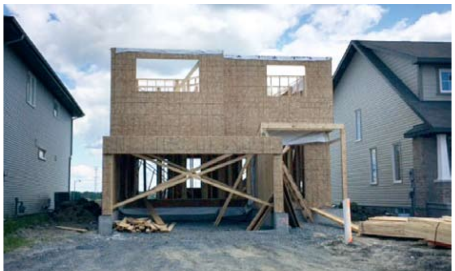
From top: June 20 - The hole that's been dug for the foundation; July 4 - Walls start to go up; July 9 - Second floor is up.
